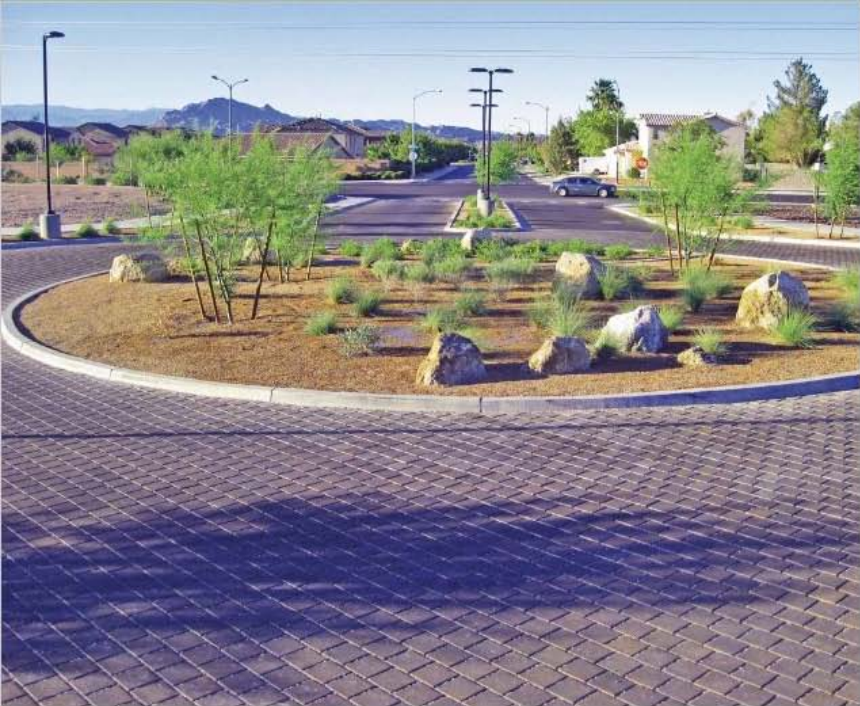
Above: Sustainable stormwater management includes permeable vehicular pavers for the "ceremonial" entry roundabout, which focuses views into the pedestrian plaza. Parking, however, is adjacent to the plaza. The infrastructure directs runoff to the onsite natural arroyo before continuing to the Las Vegas wetlands.
